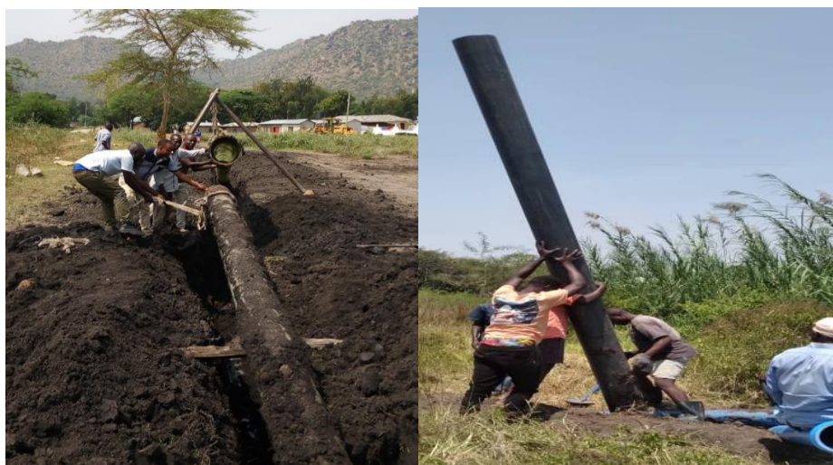
Plate 1- MUWASA Workers Replacing Burst Water Pipes in a Distribution Line
